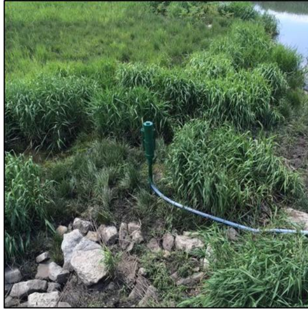
Figure 6. The onshore PVC Unit that houses the logging end of the pressure transducer.
