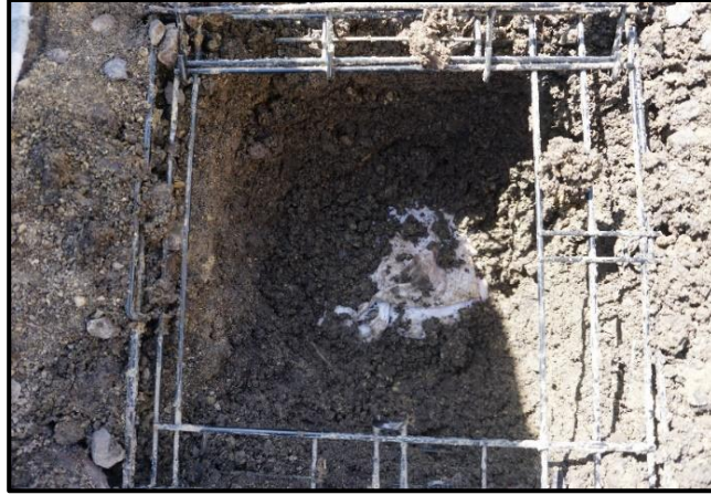
Figure 17. Top portion of specimen B visible during the two-month excavation.
