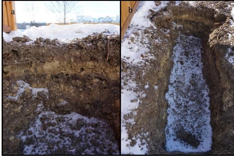
Figure 4. Stratigraphy and layout of the trench: a) Soil stratigraphy after the trench was completed; b) Layout of the constructed trench.
