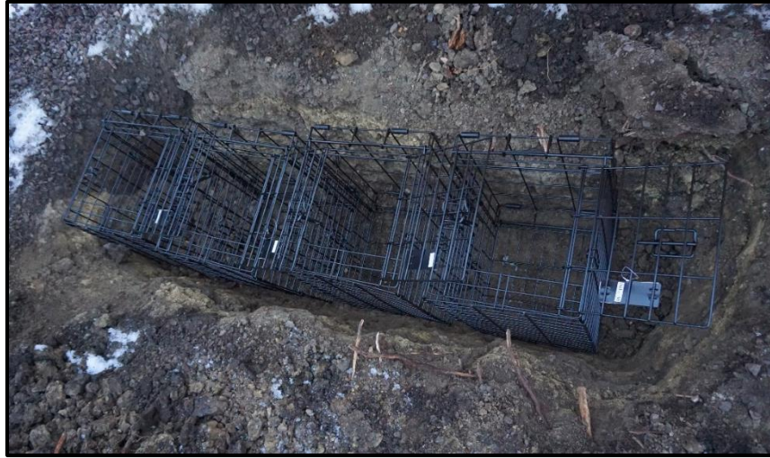
Figure 6. Cages 1-4 (18"x12"x14") within the constructed trench.
