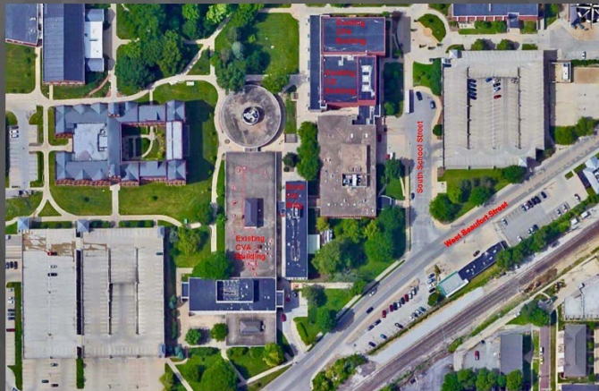
Existing Wonsook Kim College of Fine Arts (WKCF A) Complex – South ISU Quad
