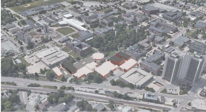
Proposed ISU CDB WKCF A Rehabilitation Project Aerial View Looking Northwest
